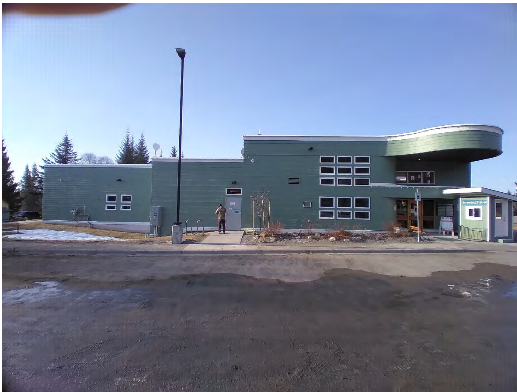
Homer Medical Center Existing Façade & Main Entry
