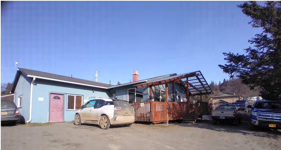
West Wing Building Existing Façade @ Main Entrance
