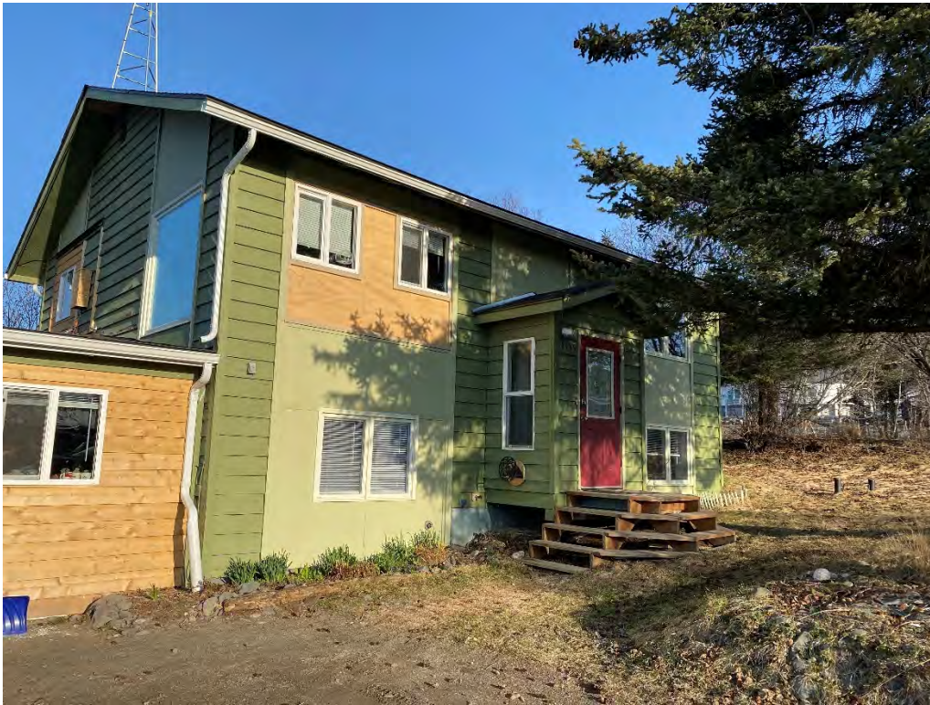
Behavioral Health Building Existing Entrance
