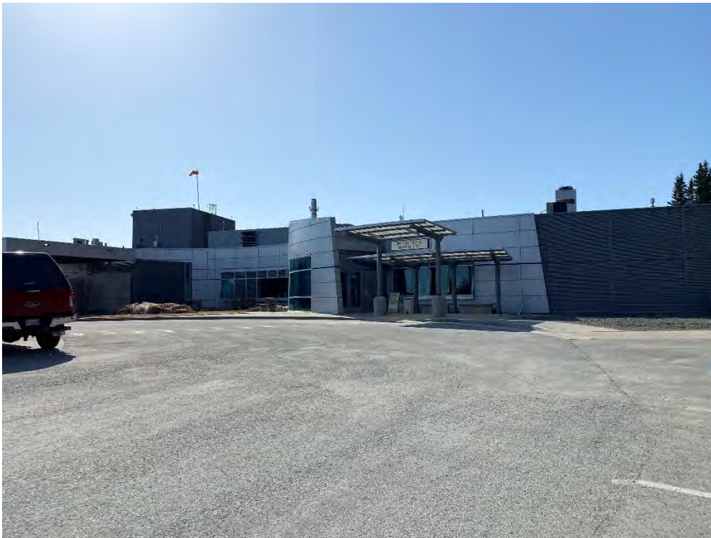
SPH Existing Façade@ Main Entrance
