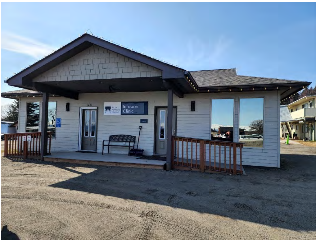
Infusion Center Existing Façade @ Main Entrance
